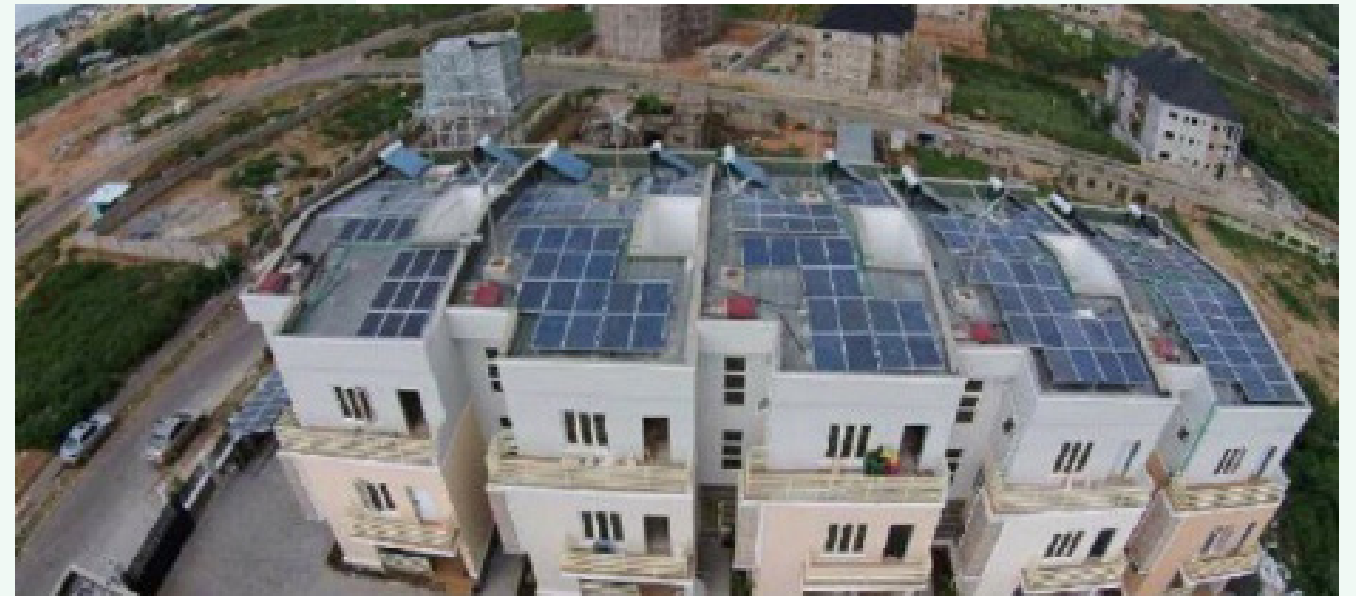
40kW off-grid solar-wind hybrid system for a block of apartments in Abuja
